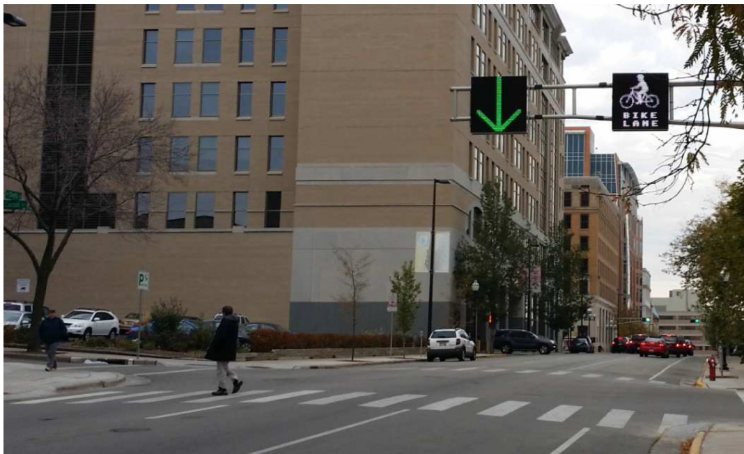
Figure 12: Dynamic Overhead Floating Bike Lane Sign (Peak-Period Condition)
