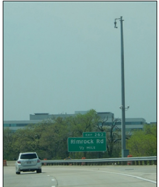
Figure 6: WisDOT Freeway CCTV Camera
