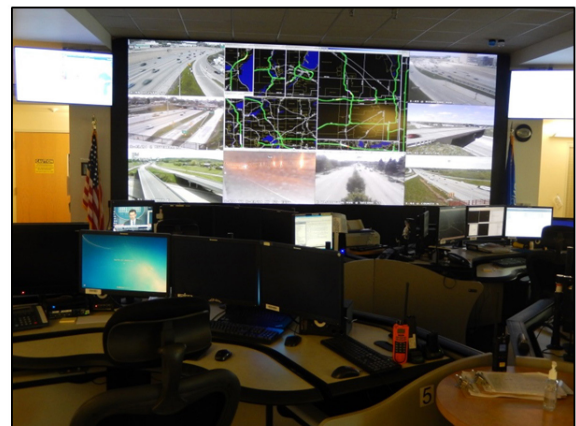
Figure 33: WisDOT STOC Control Room Video Wall
