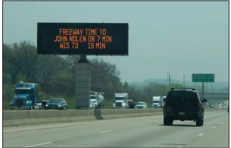
Figure 8: WisDOT Freeway Dynamic Message Sign
